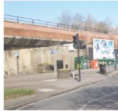
View of market area as existing with railings, concrete planters without
